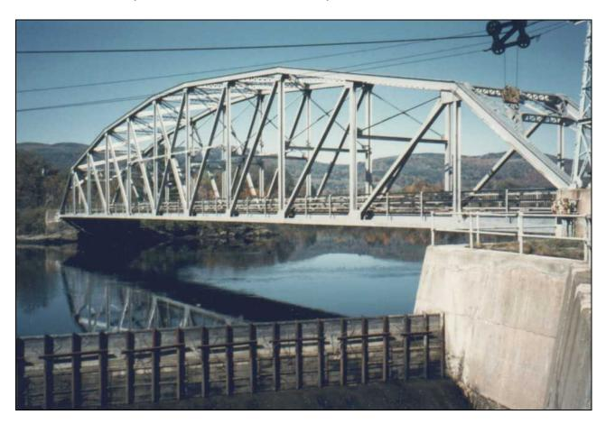
This 305-foot-span thru Pratt Steel truss bridge that connects Monroe, NH to Barnet, VT was posted for a 10-ton-weight restriction and required an extensive rehabilitation to carry legal loads.
